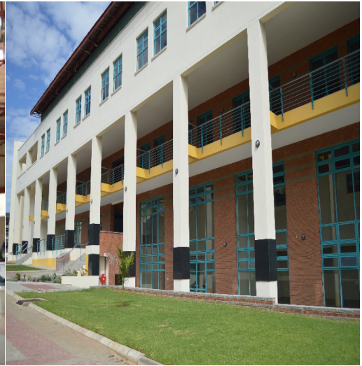
NUST Technovation Centre Block B
