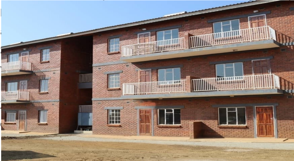
Dzivarasekwa Civil Servants Flat
